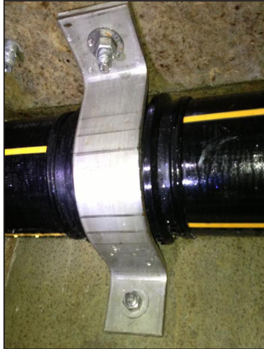
RESTRAINT FITTING
