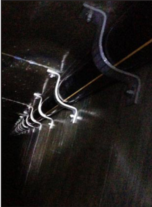
HORIZONTAL PIPE SUPPORTS
