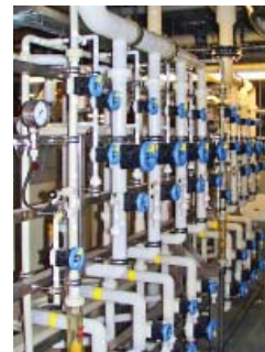
Purad® ultra high purity PVDF piping and diaphragm valves by Asahil America
